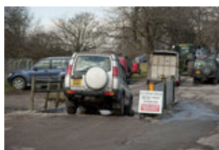
Wheel wash je021712053.jpg
