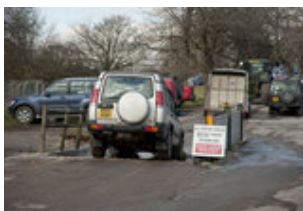
Wheel wash je021712053.jpg
