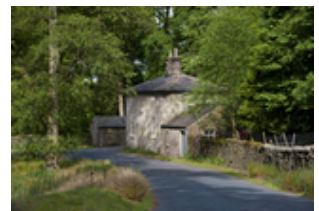
Tower Lodge je050220120013.jpg
