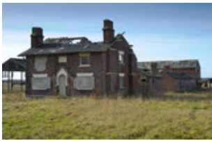
Derelict buildings je021712151.jpg
