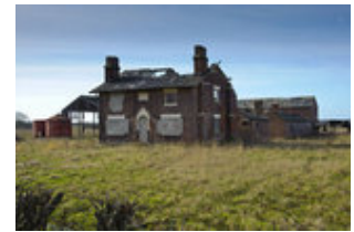
Derelict buildings je021712150.jpg
