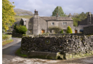
Old Farmhouse JE141112F079.jpg
