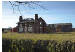
Derelict buildings je021712149.jpg
