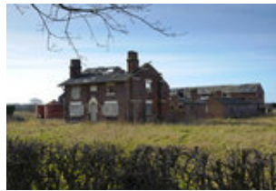
Derelict buildings je021712149.jpg
