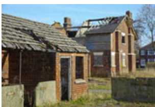
Derelict buildings je021712155.jpg
