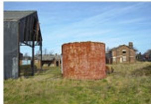
Derelict buildings je021712153.jpg
