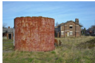
Derelict buildings je021712152.jpg
