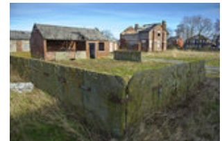
Derelict buildings je021712154.jpg
