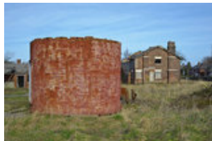
Derelict buildings je021712152.jpg
