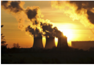
Power Station je090411039.jpg
