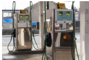
Filling station je070812019.jpg
