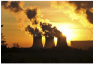
Power Station je090411039.jpg
