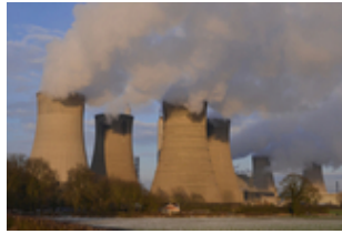
Power station JE011513155.jpg
