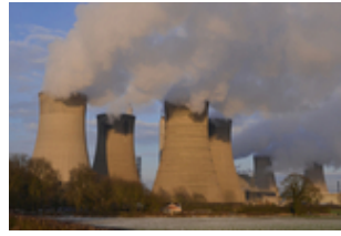
Power station JE011513155.jpg
