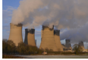
Power station JE011513155.jpg
