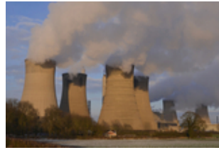
Power station JE011513155.jpg
